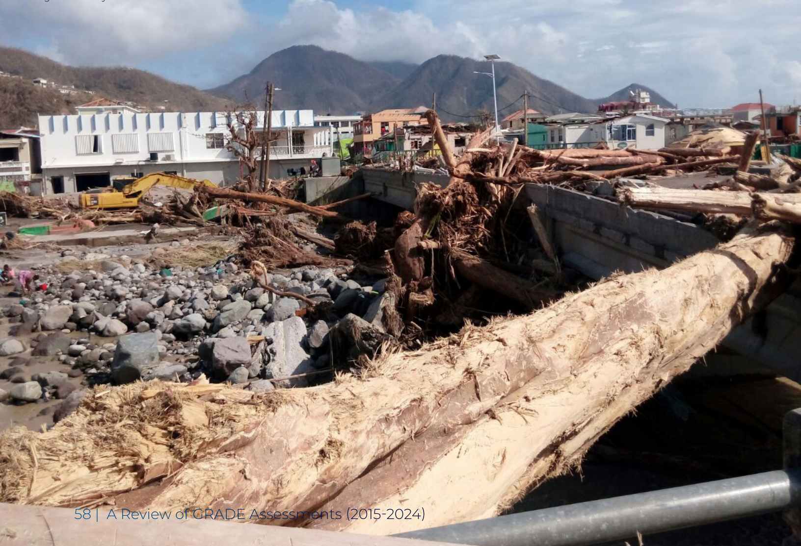
Damage caused by 2017 Hurricane Maria in Dominica. Photo Credit: World Bank
