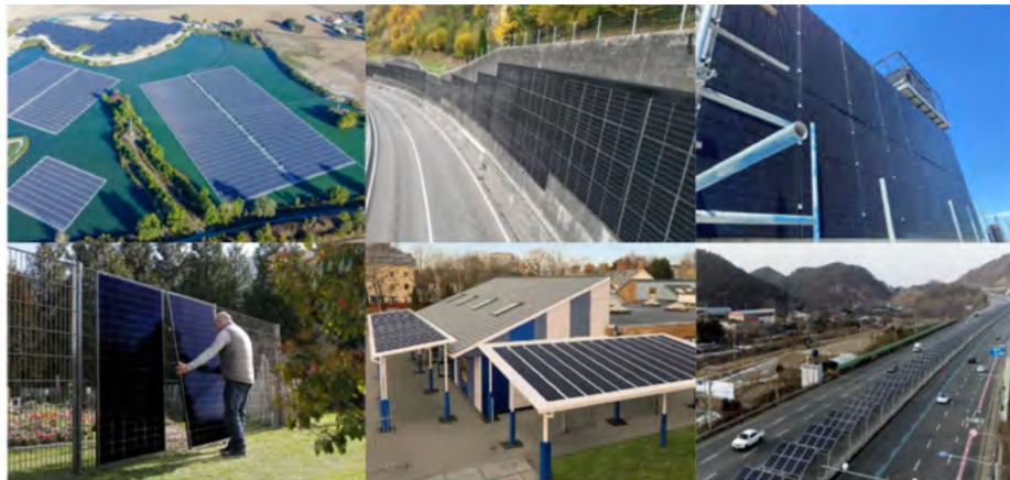
Fig 2.1. Installation of floating solar PV, road walls, building walls, fences, roofs, and canopies.
